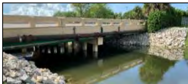
North Side of North Bridge View Looking South
