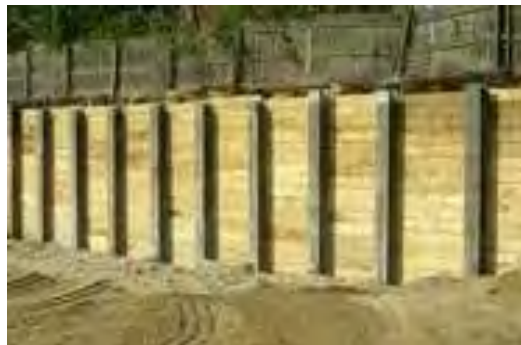
Example: H-Piles w/Lagging Boards
