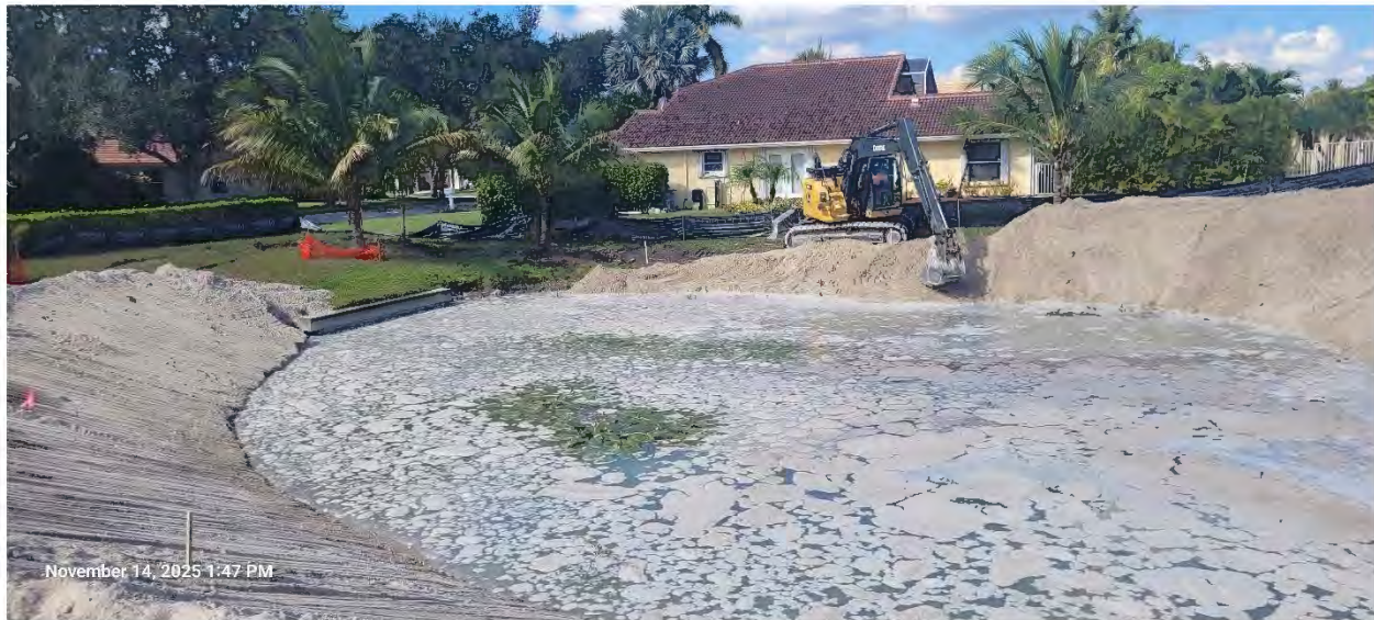
Figure 1 – Pond bank regrading
